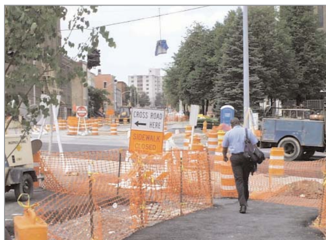
ADA compliant channelization to a pedestrian crossing was provided at N. Pearl and Clinton Street.
