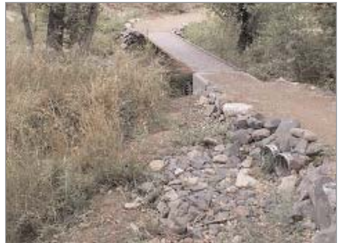
The Granite Creek bridge takes advantage of an existing sewer pipe as its foundation.
