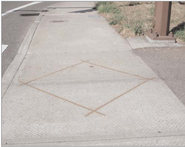
A bicycle-activated Signal Loop Detector.
