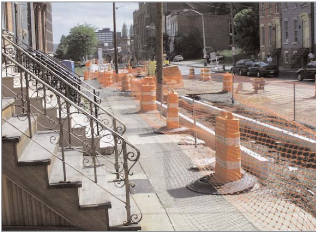
Cane-detectable fences were installed beside sidewalk widening and new curb work on N. Pearl Street.
