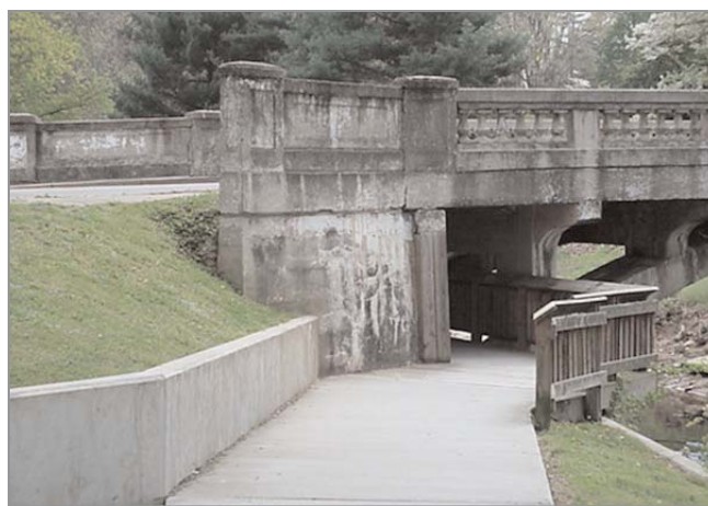
The pedestrian trail bridge utilizes the space beneath the Eighth Street roadway bridge at Four Pole Creek.
