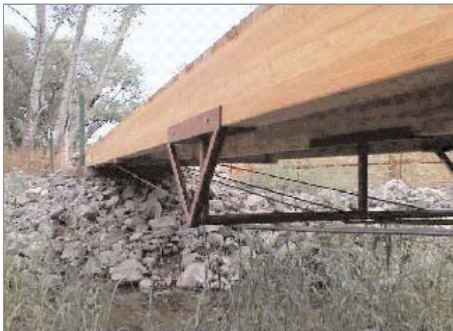
The Miller Creek permanent bridge tension frame was used to steady the bridge for pedestrians and bicyclists
