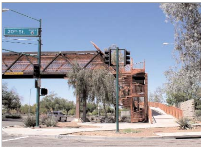
New ramps, spiral staircases, and footings were constructed to comply with ADA standards.
