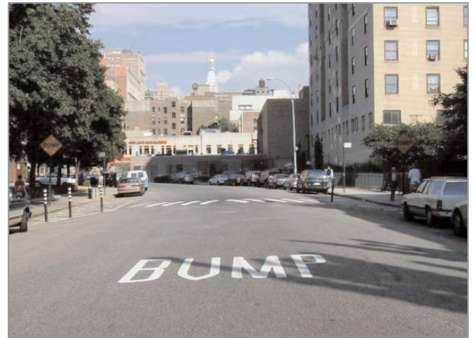
24th Street was narrowed at the crossing point to complement the speed table.
