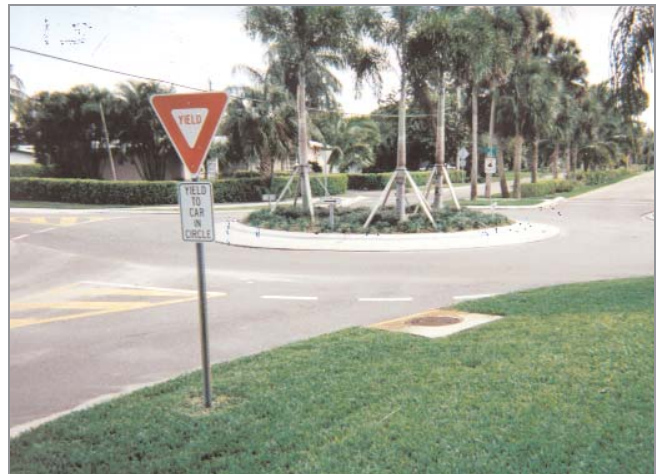
Median island and intersection roundabouts were installed on 7th Avenue.
