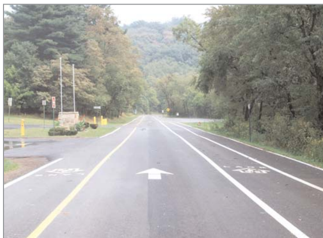
Striping of three travelways—center lane for one-way vehicle flow, a parallel flow bicycle lane on the right, and a contra-flow bicycle lane on the left.
