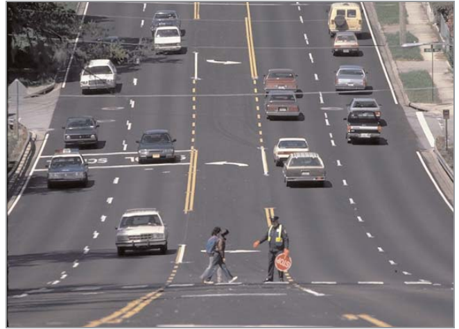
Wide multilane roadways without adequate crossing islands create an unsafe environment for many pedestrians.
