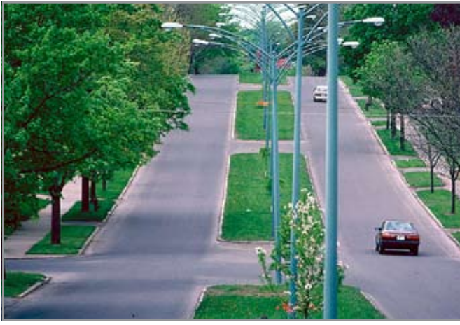
Raised medians provide another option for locating lighting on this shared roadway.
