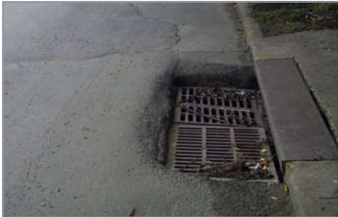
Below-grade drain grates create hazards for bicyclists.
