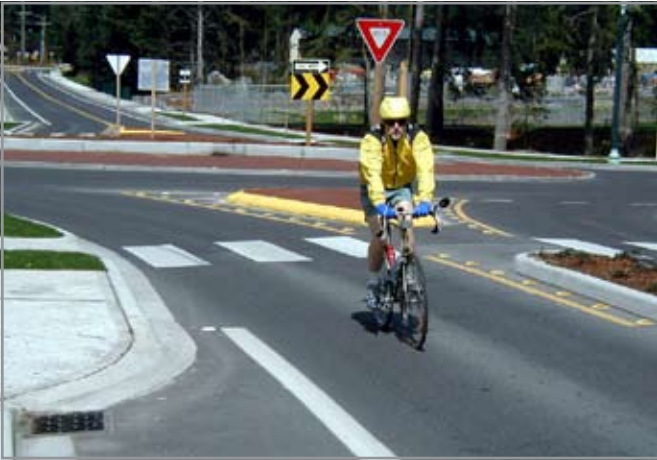
Splitter islands and narrow curb radii slow speeds approaching the roundabout.
