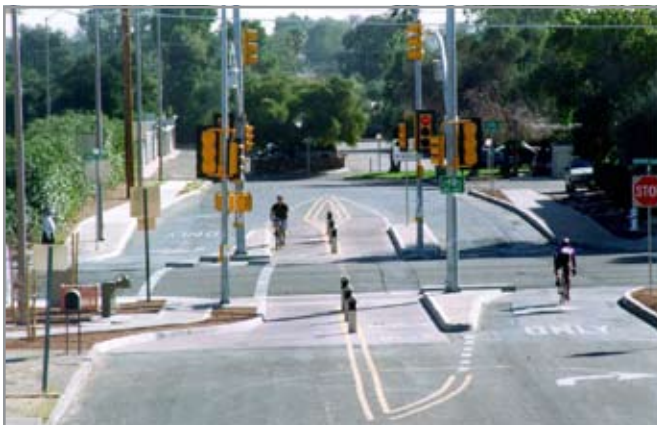
Diverter and toucan signals help create a bicycle boulevard in Tucson, AZ.
