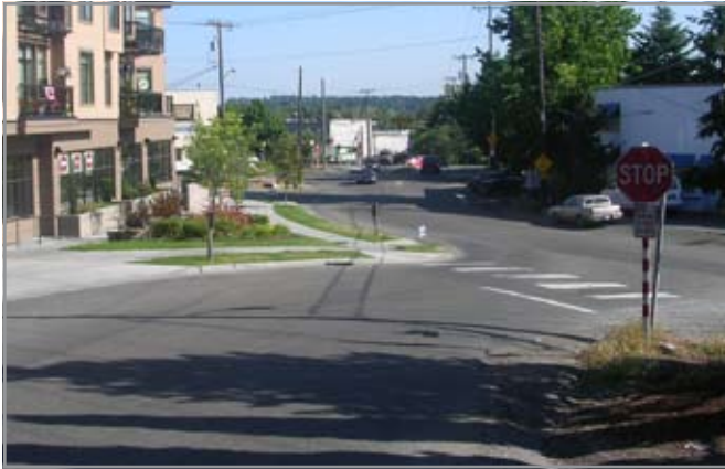
Realigning skewed or obtuse-angle intersections improves sight angles for intersecting roadways.
