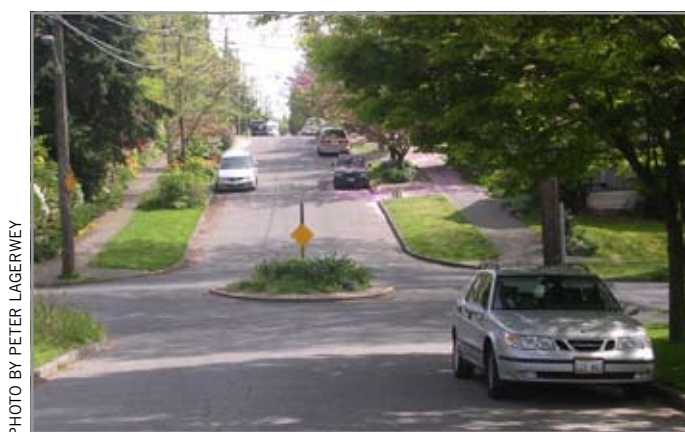
Motor vehicles must slow to navigate through mini circles such as this one in a Seattle, WA, neighborhood.
