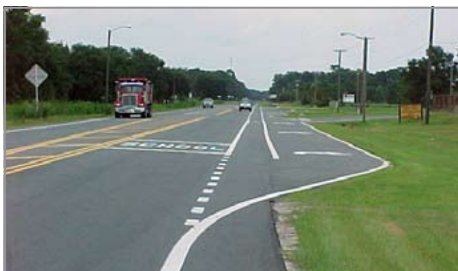
Bike pocket striped to the left of a right-turn lane aids through bicyclists using a paved shoulder facility.
