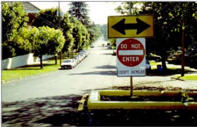
A partial closure limits cut-through traffic but allows bicyclist access.
