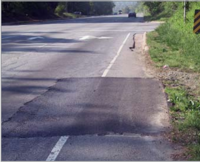
Sunken pavement patch and shoulder drop-off to below-grade drainage grate contribute to bicyclist discomfort and possible hazards for bicyclists.
