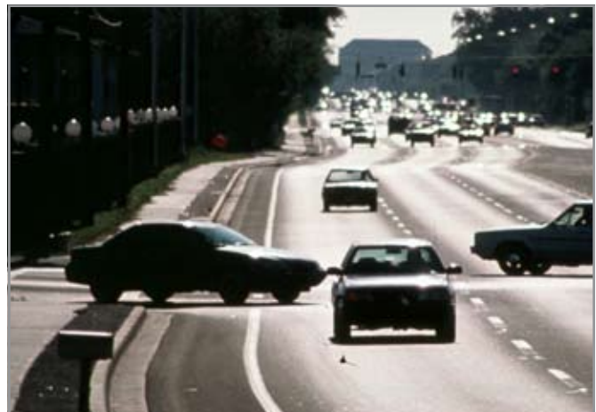
Good sight distance helps reduce the potential for conflict between the vehicle emerging from the driveway and a bicyclist in the bike lane.
