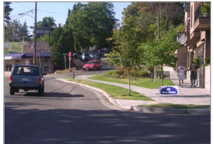
Tighter curb radii at obtuse angle corners forces slower motorist turns. (Seattle, WA)
