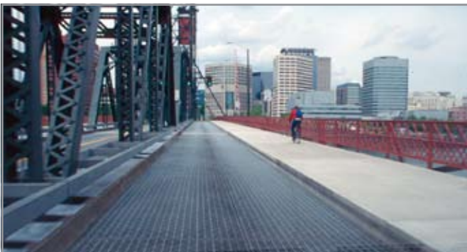
This cantilevered, shared-use path was added to the Steel bridge in Portland, OR.
