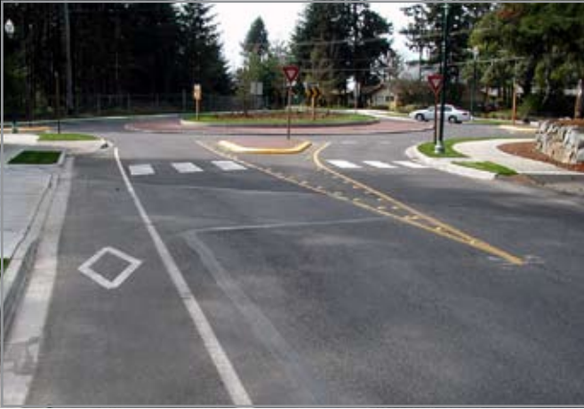
Bike lanes should be discontinued before roundabouts.
