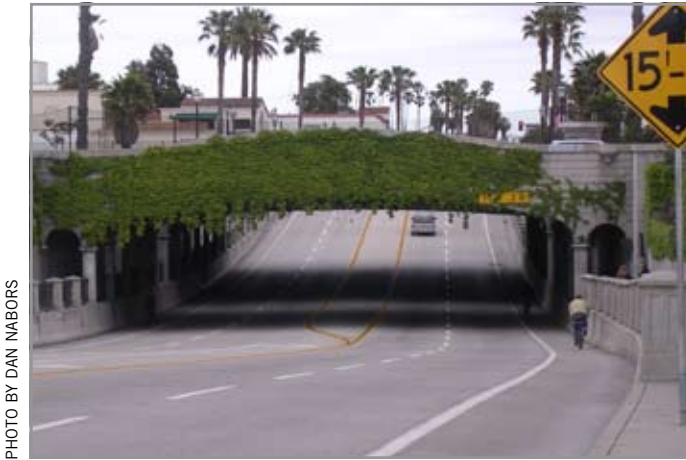
State Street underpass with bike lanes, Santa Barbara, CA. Sidewalk is elevated above the roadway.
