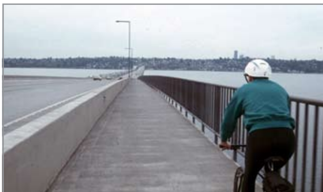
Extra width, concrete barrier, and outside railing protect bicyclists from strong wind gusts. (Seattle, WA)
