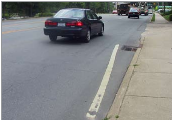
Short term solution of pavement marking highlights the hazard until unsafe drain grates can be replaced or repaired.
