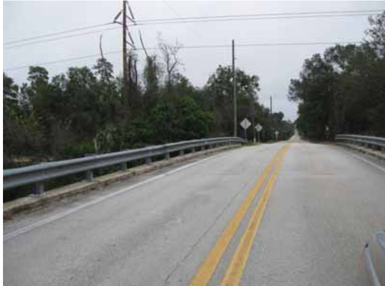
Figure 3 - Restricted shoulder on existing bridge
