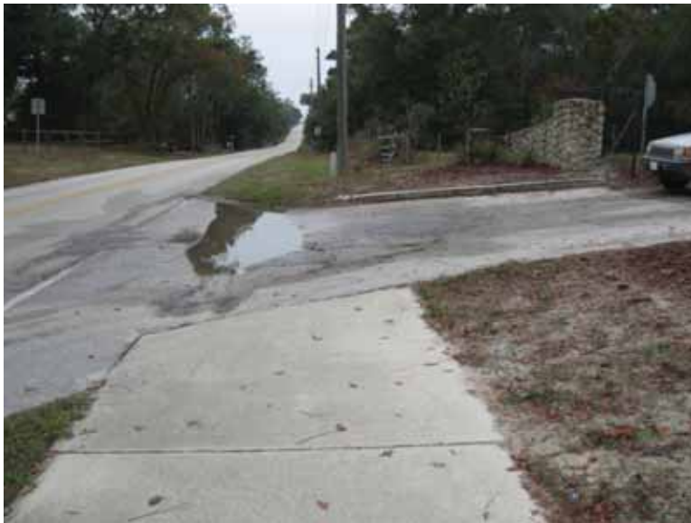
Figure 7 - Entrance to Valentine Park to be reconstructed to mitigate grades and drainage issues
