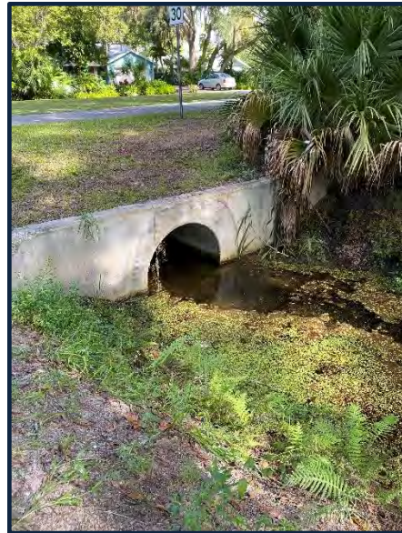
FIGURE 7: EXISTING 54-INCH OUTFALL #2 EAST OF WESTWOOD AVENUE
