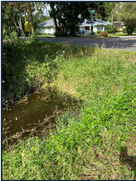
FIGURE 6: EXISTING 48-INCH OUTFALL #1 AT CLARENDON AVENUE
