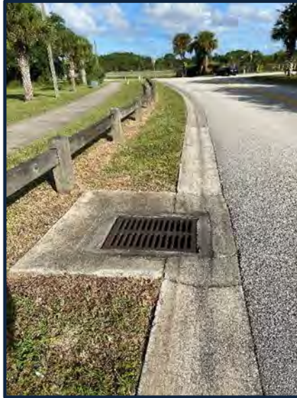
FIGURE 5: EXISTING TYPE C INLET ALONG SUNSET DRIVE
