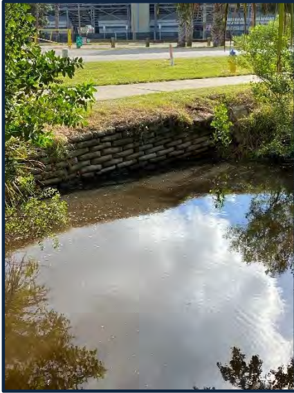
FIGURE 8: EXISTING HEADWALL & CROSS DRAIN #1 AT SUNSET DRIVE
