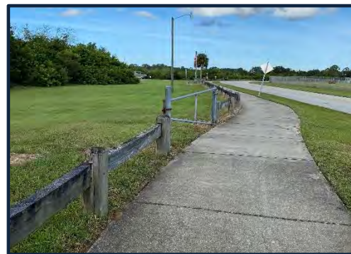
FIGURE 14: EXISTING FENCE & GATE ALONG SUNSET DRIVE LOOKING NORTH
