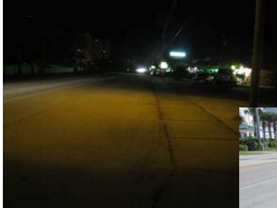
Limited Roadway Lighting Effectiveness
