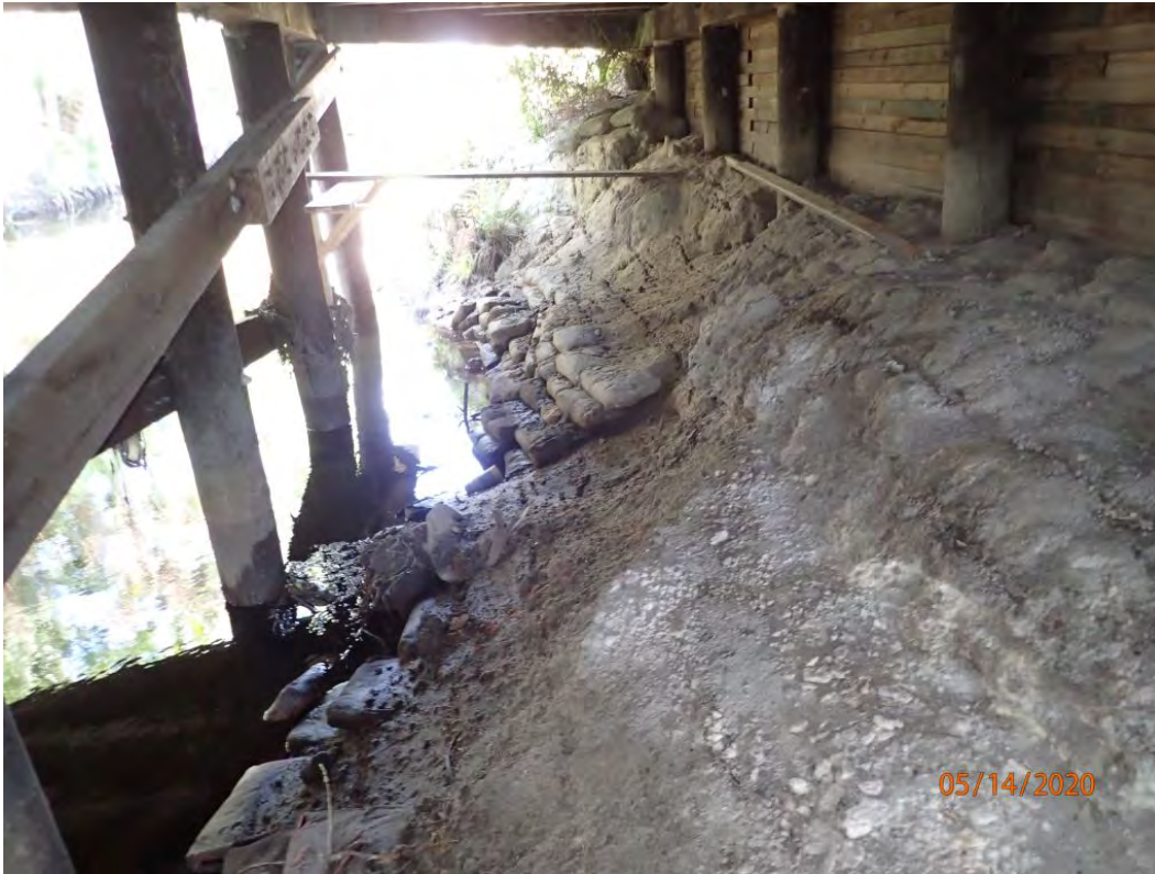
Photo 3: Element 8290: Showing channel bank erosion and displaced rip rap bags.
