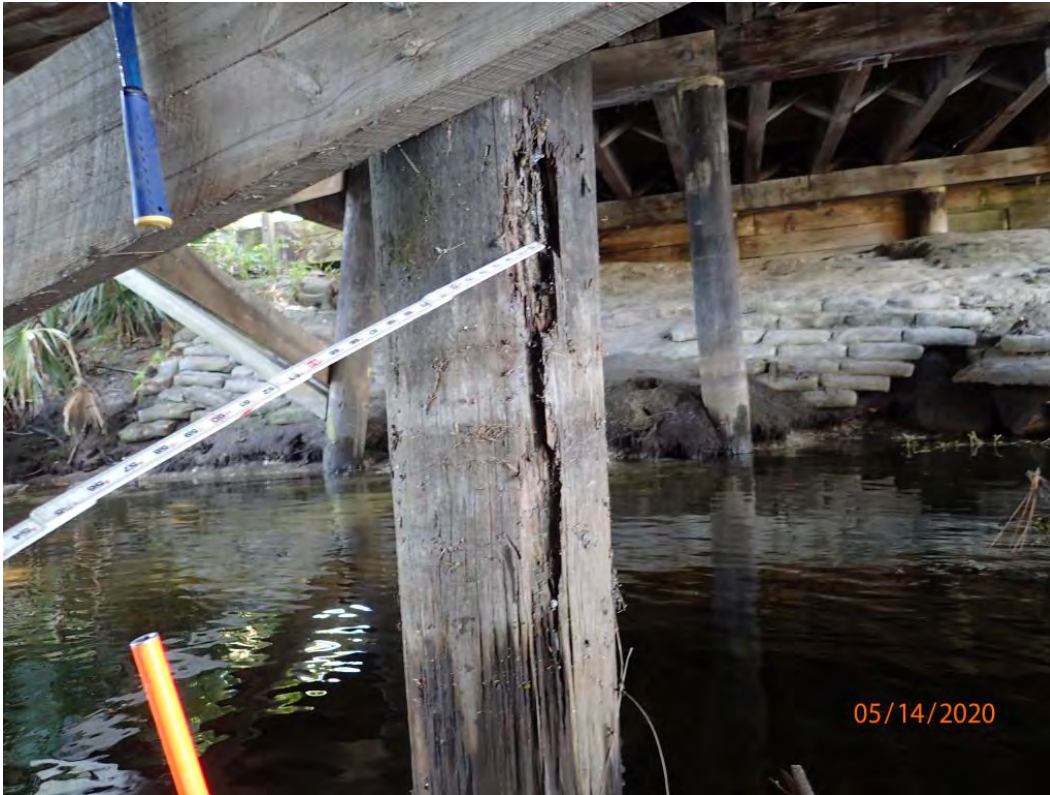
Photo 7: Element 228: Showing heavy decay at Pile 3-3.
