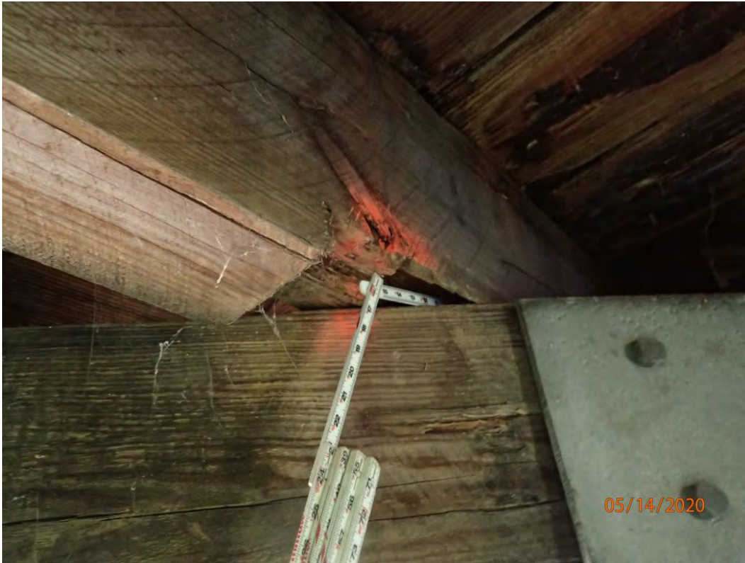
Photo 9: Element 111: Showing decay at timber stringer 4-19.
