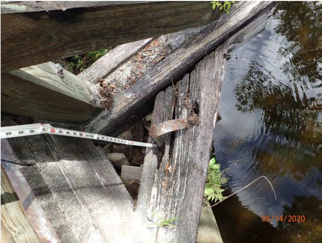
Photo 8: Element 235: Showing heavy decay at Bent 4 cap and horizontal brace.
