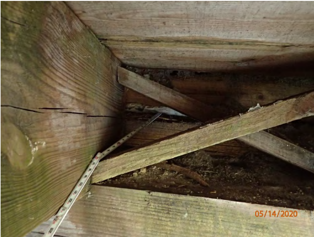
Photo 4: Element 8476: Showing fill migration and decay at Abutment 1 backwall.
