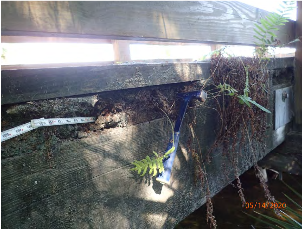
Photo 1: Element 31: Outer ends of transverse timber deck are wet, soft, and decayed.
