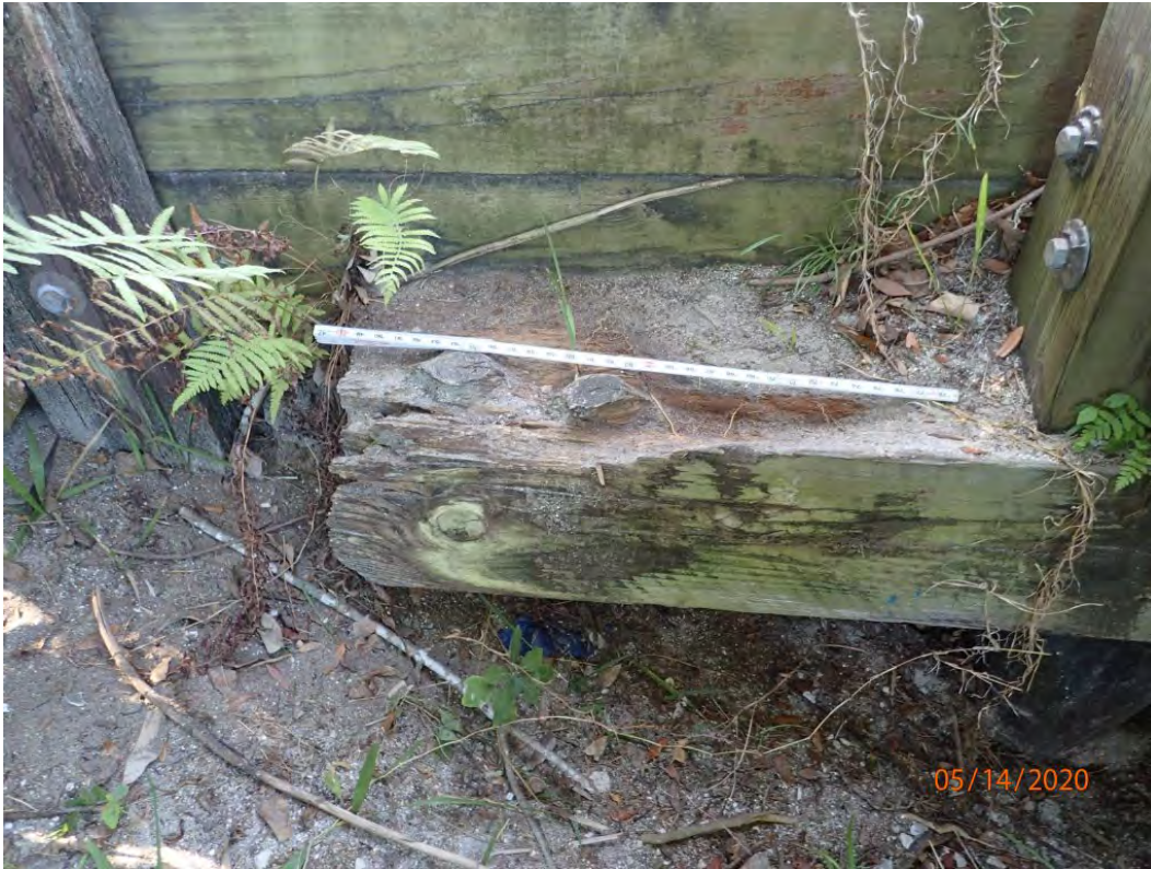
Photo 5: Element 216: Showing heavy decay at east end of Abutment 1 cap.
