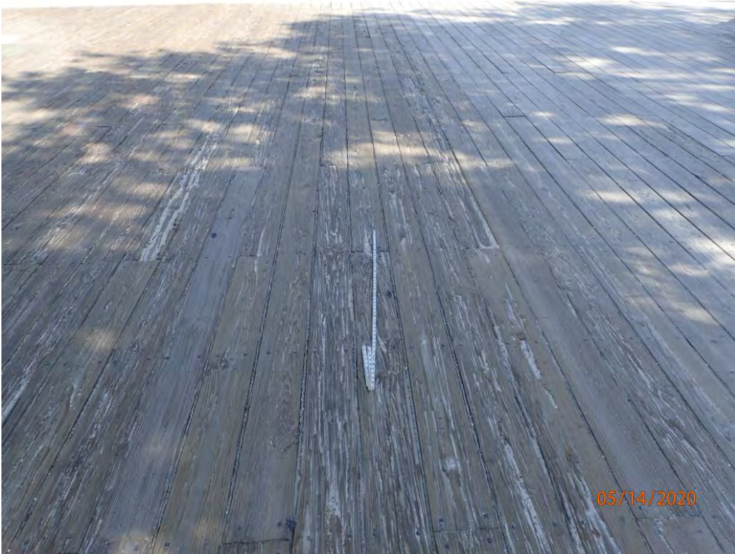
Photo 2: Element 31: Showing weathered and checked timber running boards.
