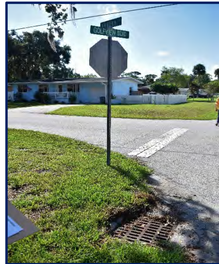
Figure 10: Drainage Inlet at Aurora Street to be relocated
