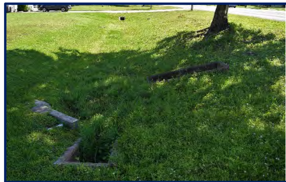
Figure 8: Existing U-Type Endwalls and Straight Endwalls along Big Tree Road
