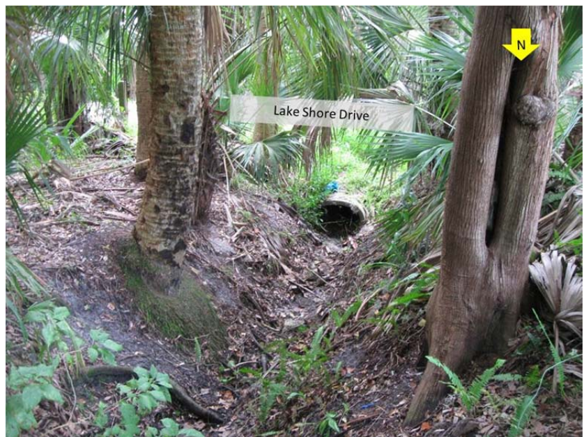
Figure 19: View of culvert under Lake Shore Drive between the Senior Center and Green Springs Park.
