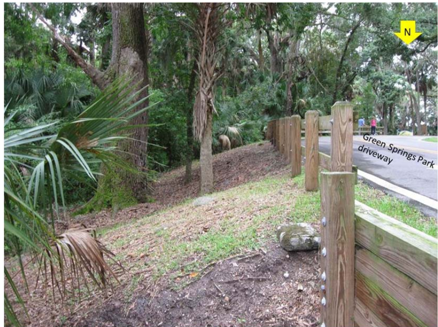
Figure 27: View of east side of Green Springs Park driveway.
