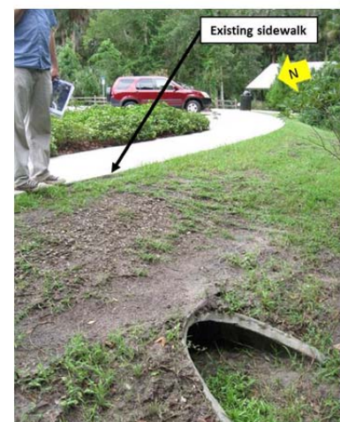
Figure 24: Mitered end section would need to be lengthened with sidewalk widening.
