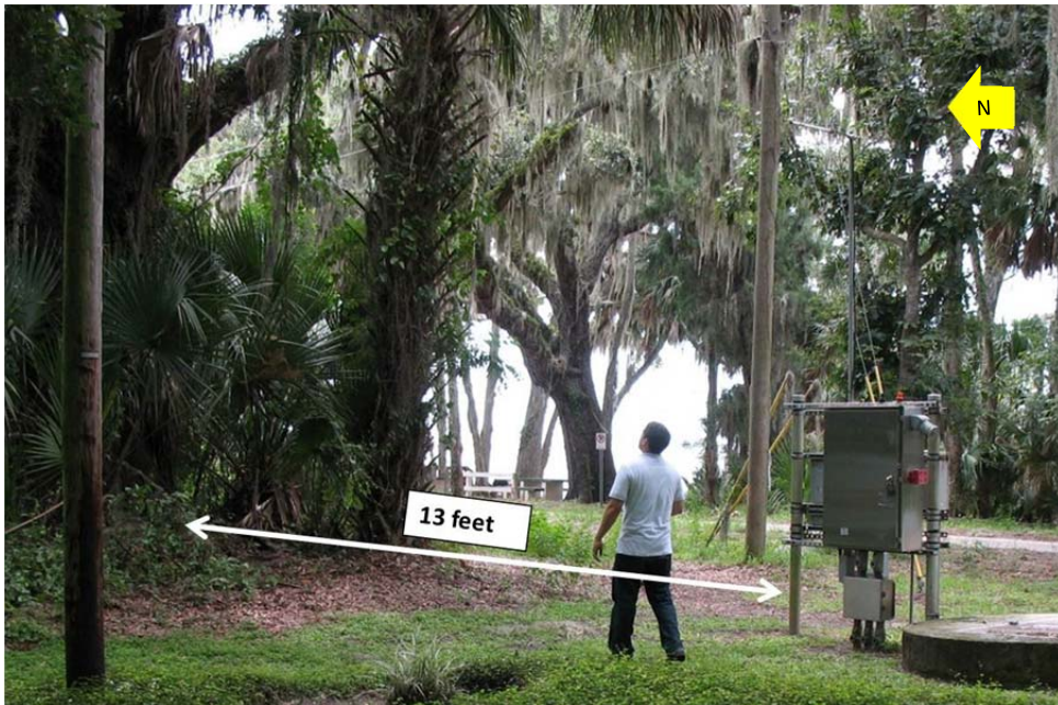
Figure 16: Limited horizontal clearance between an existing tree and lift station equipment may require a brief narrowing of the trail.
