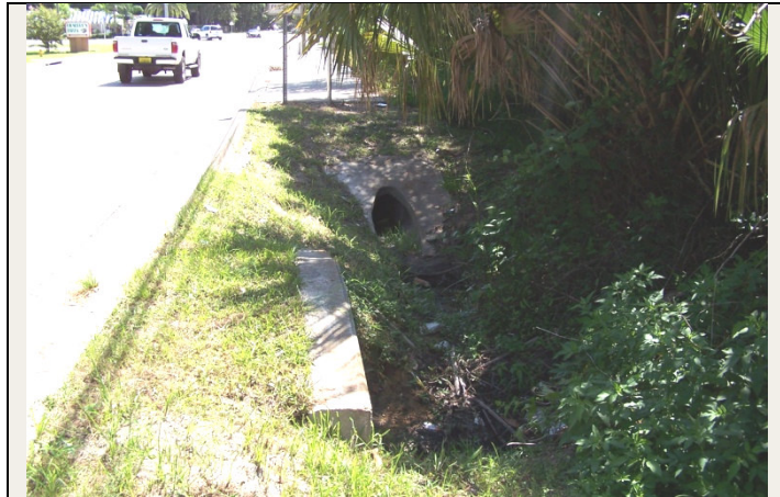
Cross drain headwalls, mitered end culvert, and small swale west of Nova Road (Looking East)
