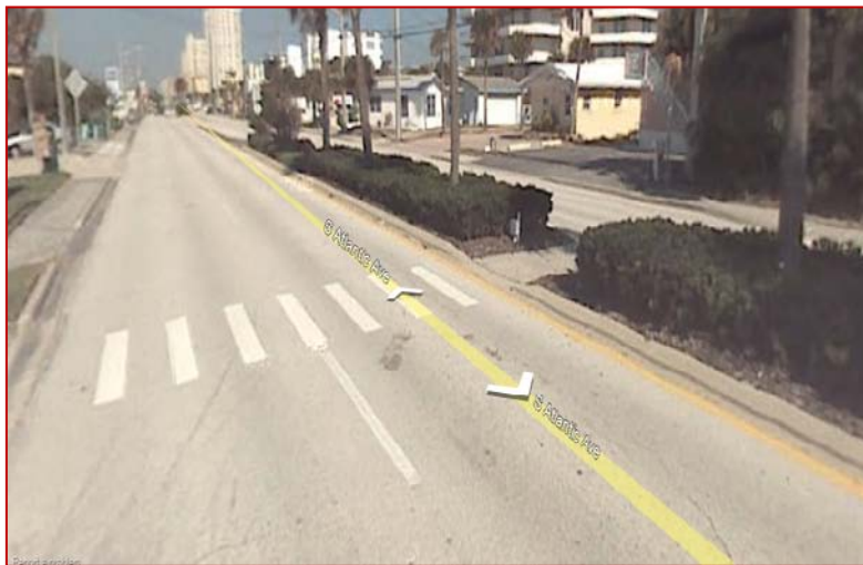
Figure 5: Picture of a Median Refuge Island on S Atlantic Avenue between Dahlia Avenue and Phyllis Avenue (source: Google Maps)
