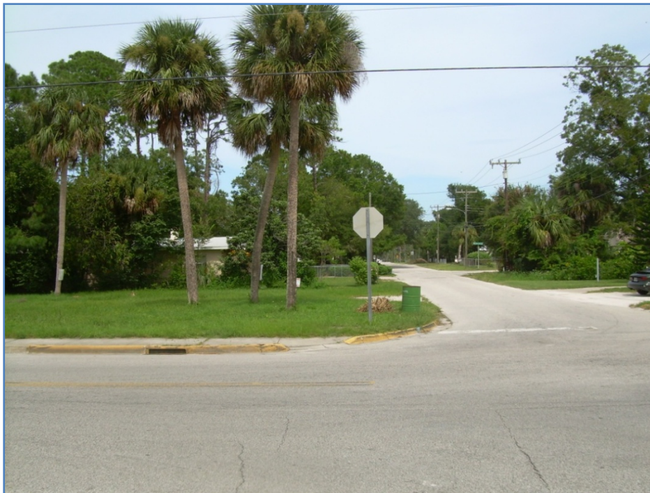
Northeasterly view along Fremont Avenue at the intersection of Dr. Martin Luther King Jr. Boulevard. An existing 5-foot wide concrete sidewalk with access ramp is located along the east side of Dr. Martin Luther King Jr. Boulevard. No pedestrian cross-walk striping has been provided across Fremont Avenue. A pedestrian cross-walk will also be required across Dr. Martin Luther King Jr. Boulevard.
