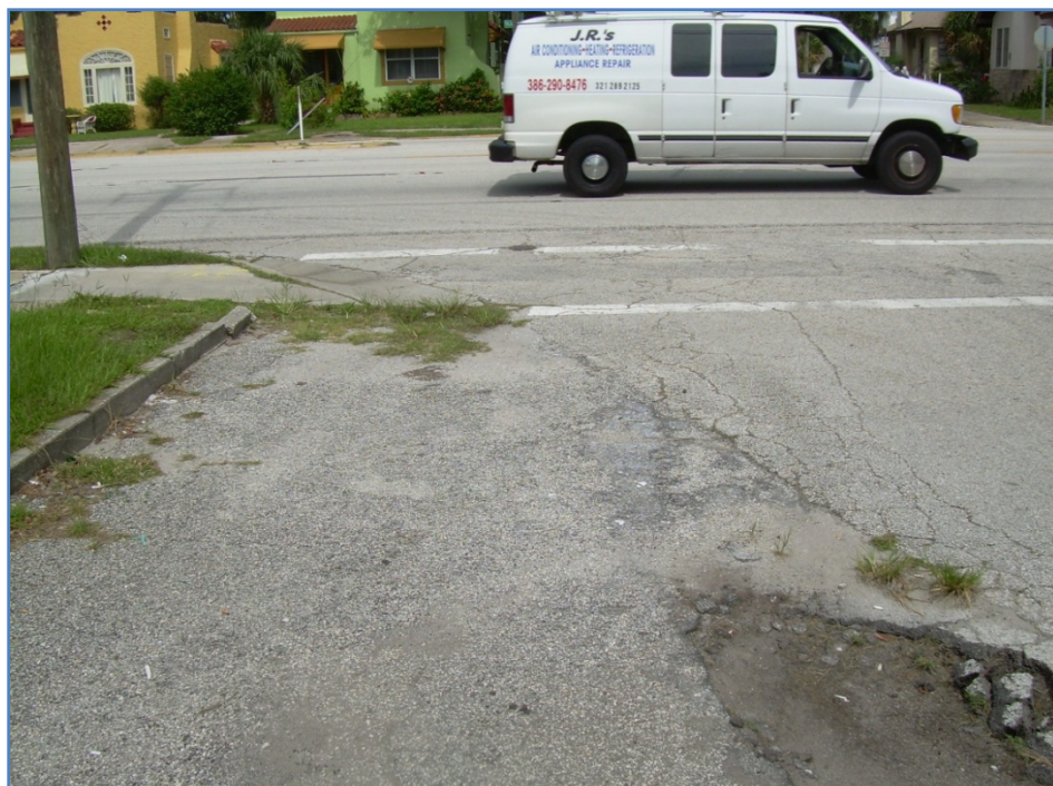
Northerly view along Ridgewood Avenue (U.S. 1) showing the existing 5-foot wide concrete sidewalk with access ramp. Existing asphalt paving within the right-of-way adjacent to the hotel as shown below.
