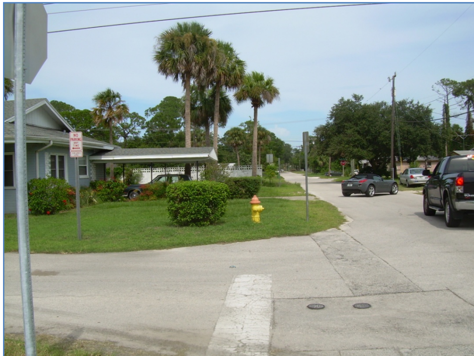
Northeasterly view along Fremont Avenue at the intersection of School Street. The right-of-way is located between the fire hydrant and the landscape hedge. Pedestrian cross-walk striping together with the traffic stop bar will be required at this intersection.
