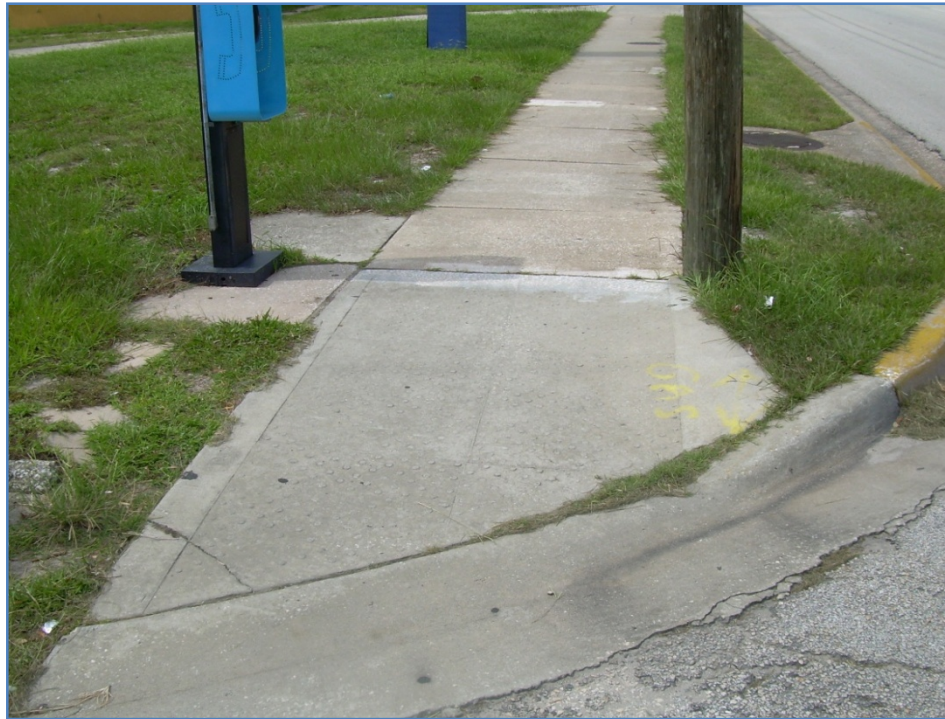
Northerly view along Ridgewood Avenue (U.S. 1) showing the existing 5-foot wide concrete sidewalk with access ramp. Existing asphalt paving within the right-of-way adjacent to the hotel as shown below.
