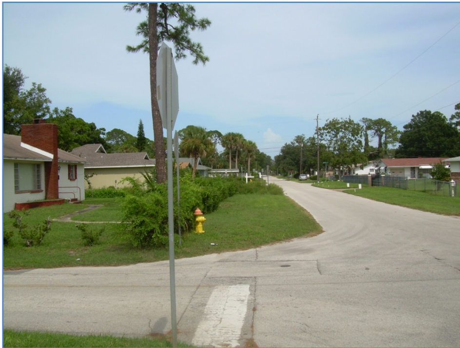
Northeasterly view along Fremont Avenue at the intersection of Vernon Street. The right-of-way is located between the fire hydrant and the landscape hedge. Pedestrian cross-walk striping together with a traffic stop bar will be required at this intersection.
