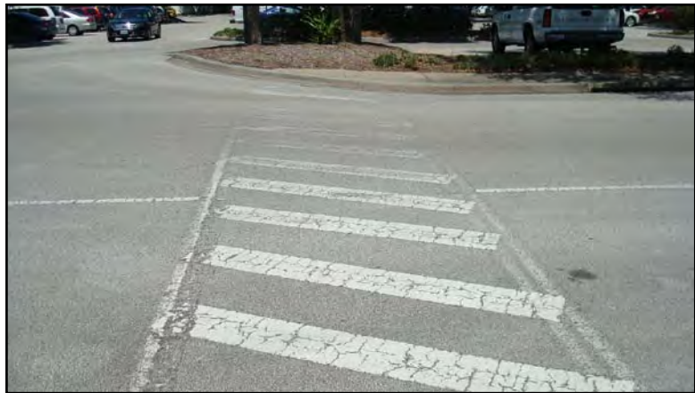
Illustration 12 Faded crosswalk markings
