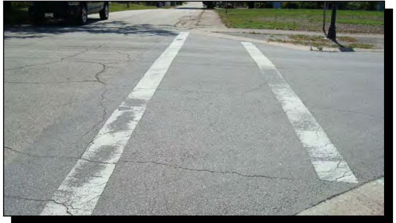
Illustration 9: Faded pavement markings on at the intersection of Ridgewood Avenue and Tomoka Avenue
