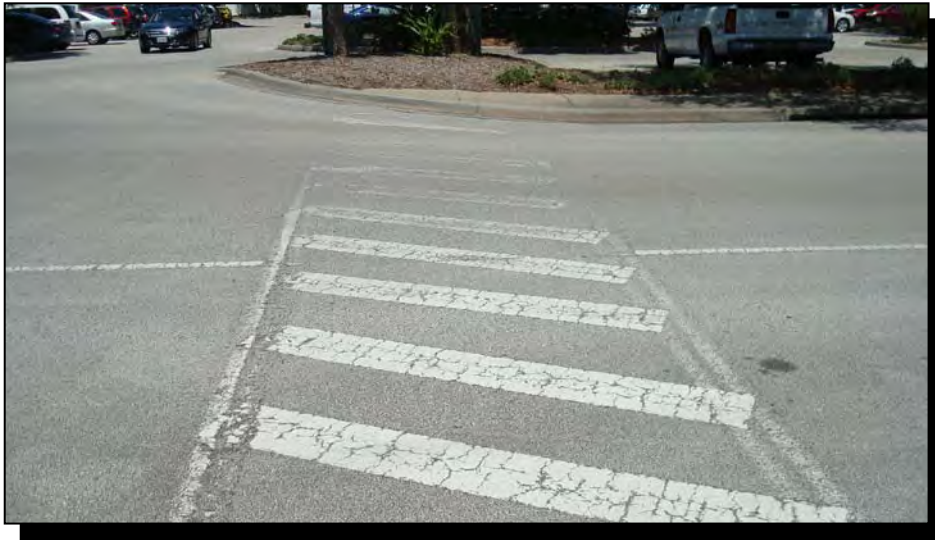
Illustration 7: Faded pavement markings on Eileen Butts Street that connects the sidewalk to the City Hall/Library parking lot
