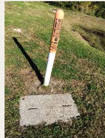
Figure 6 – Fiber optic pull box near Dunlawton Avenue
