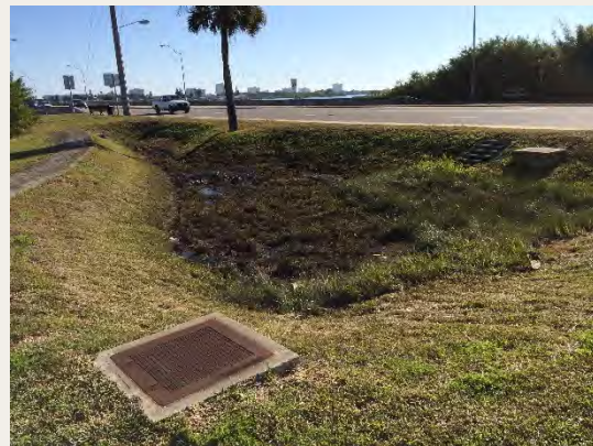
Figure 9 – Pond and underdrain inspection boxes near the intersection of Halifax Drive and Dunlawton Avenue
