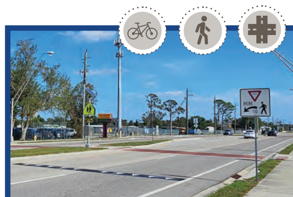
Advance Warning Signage/Markings
