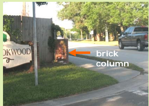
Sight distance is reduced by an unused brick column at the intersection of Brookwood Drive with Old Tomoka Road
