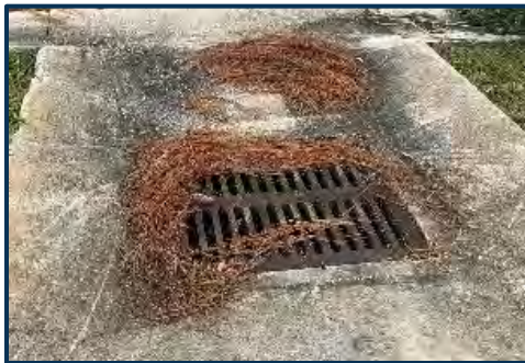
Figure 6: Type C Ditch Bottom Inlet
