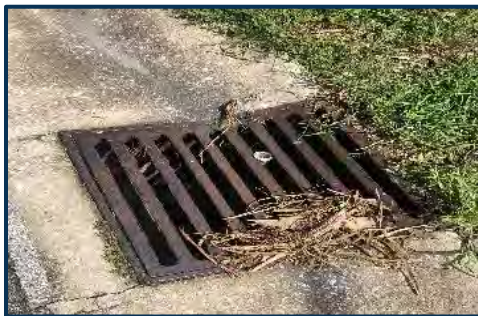
Figure 7: Gutter Inlet
