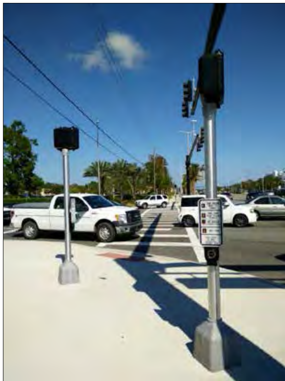
Figure 1 Accessible Pedestrian Signal devices at International Speedway Blvd and Williamson Blvd in Daytona Beach, FL
