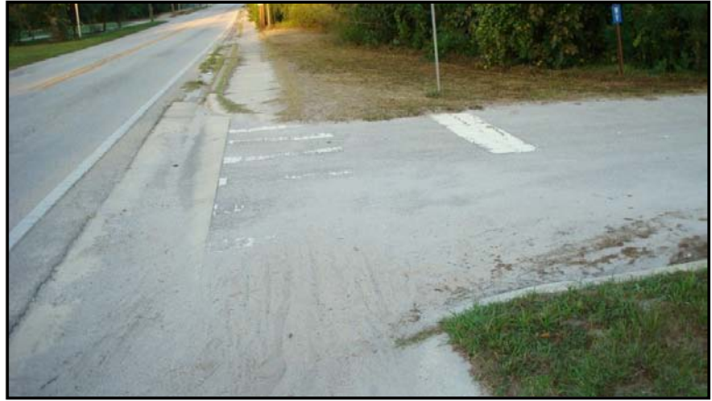
Illustration 18: Faded crosswalk markings
