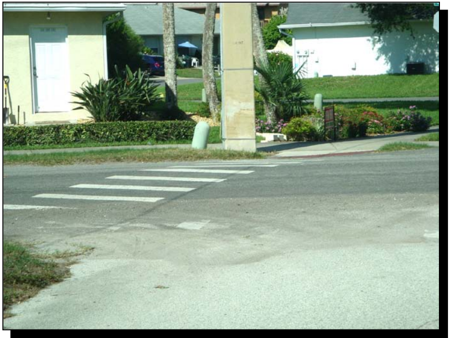
Illustration 14: Faded crosswalk markings at the intersection of Saxon Avenue and Sandpiper Street
