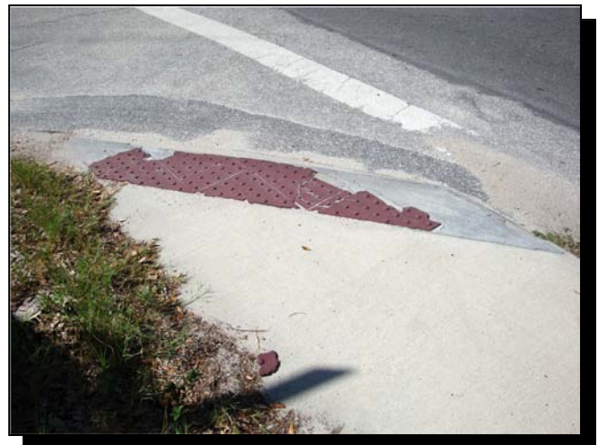
Illustrations 17 and 18: No sidewalk connection in the northeast quadrant at Saxon Drive and Mathews Avenue
