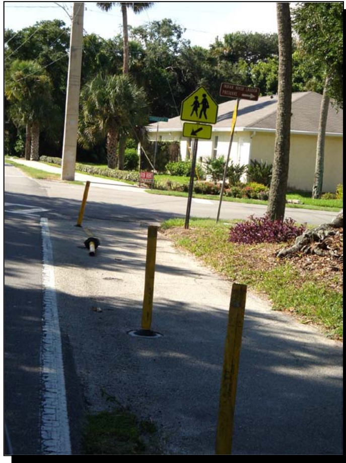
Illustration 11: Broken tubular delineator at Saxon Drive and Sandpiper Street
