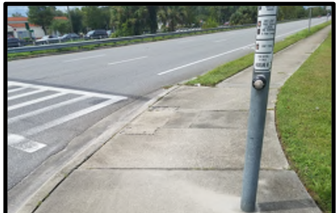
Pedestrian detector in the northeast quadrant.
