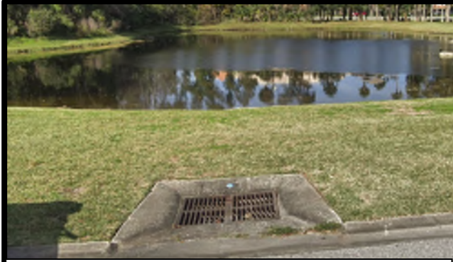
Looking northwest at the existing catch basin with concrete apron near station 14+40 (LT)
