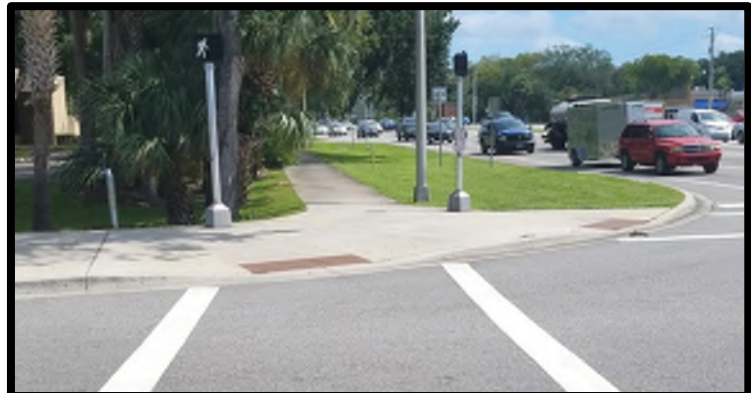
Pedestrian ramps and signal poles with detectors in the northeast quadrant looking east from the north leg crosswalk.
