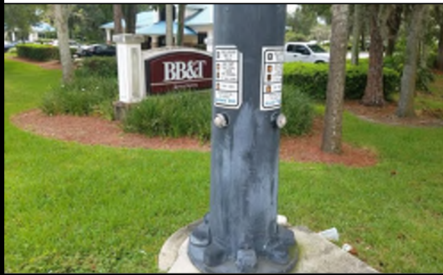
Pedestrian detectors on traffic signal mast arm in the southwest quadrant.
