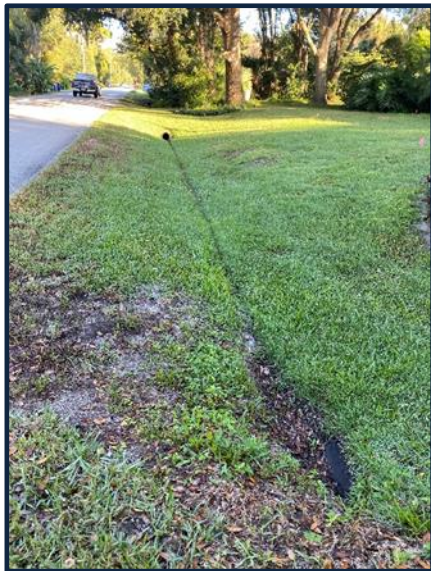
FIGURE 5: EXISTING DITCH WITH SIDE DRAIN
