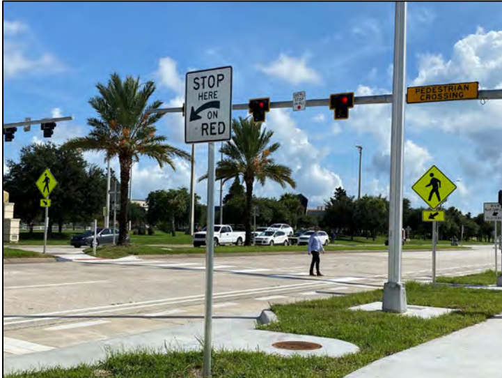
PEDESTRIAN USING NEW PHB SIGNAL AT MAINLAND HIGH
