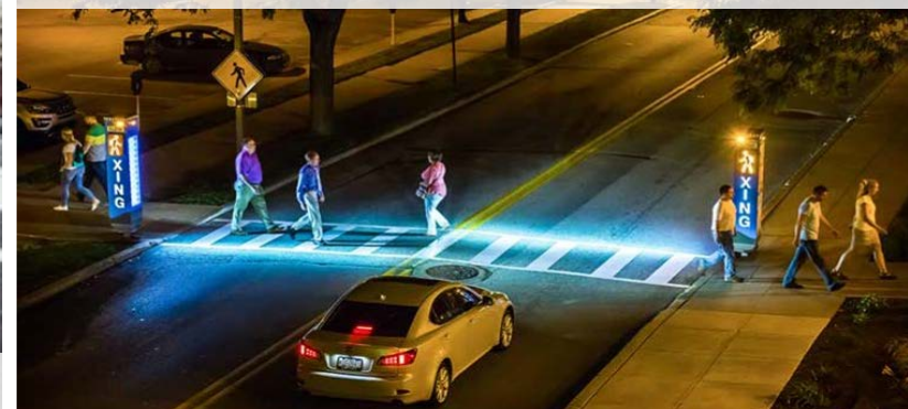
High Emphasis Pedestrian Crosswalk Lighting
