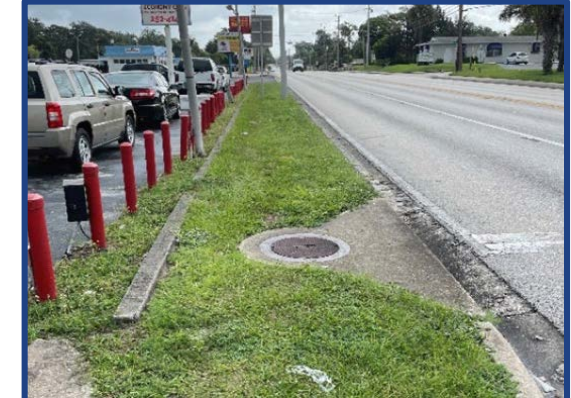
Lack of sidewalk facility
