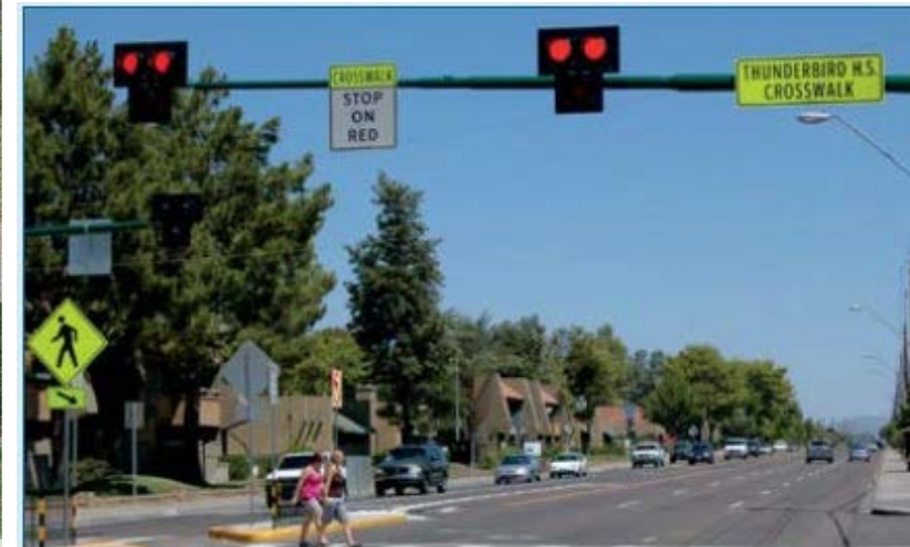
Mid-Block Crossing (with PHB)
